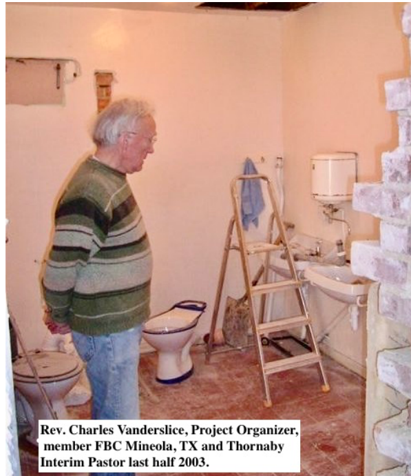
Original Toilet with too narrow entrance door and toilet too low.
